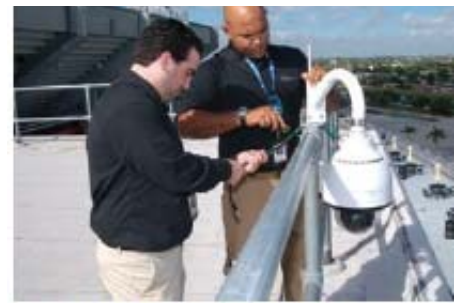
Aware Digital's Joshua Mann (left) and Adan Canuelas install one of the project's Sony SNC-RH164 high definition pan/tilt/zoom cameras. Many of the cameras are semi-permanent in that they can be easily deployed as events dictate.
